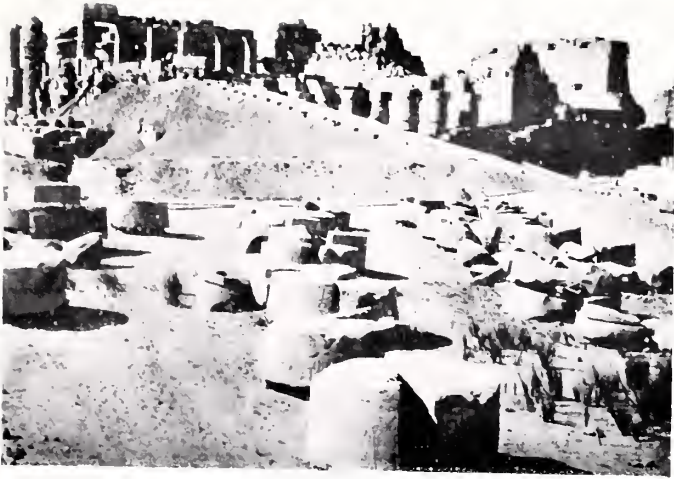
I. Inclined Plane Used in Taking Down the Columns.
